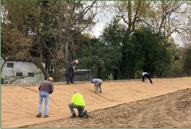
CLCF's Stew Crew Placing Erosion Matting
