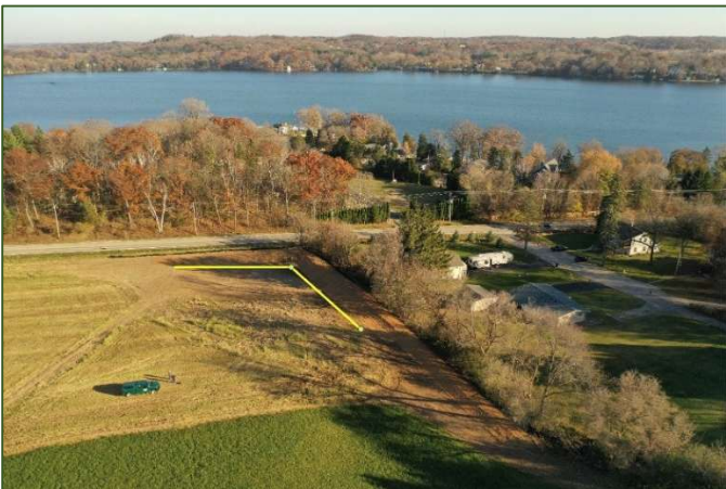
East field constructed WASCOB (yellow line) along the road and tree line. Photo courtesy of Washington County
